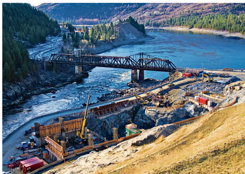
Construction of the $900 million 335-MW Waneta Expansion hydroelectric generating facility is progressing well.
